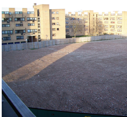
RE-USE: Recycled concrete aggregate was crushed and left on site (top right) and then used for landscaping (above).
