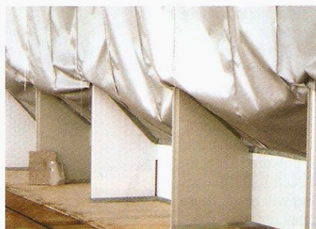
The custom-made fire curtain spanned 160m (top); curtain sections were bolted to floor angles and then stapled together (above)
