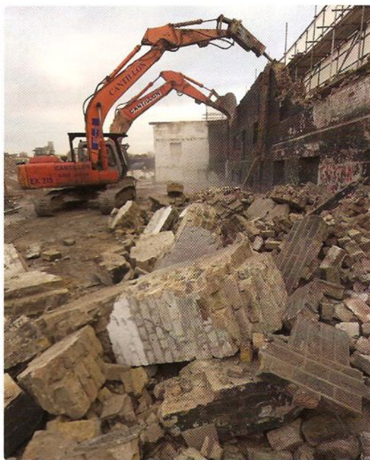
Figures 3 (right) and 4 (below): The walls of the building are carefully pulled down under close supervision and brick, stone and concrete is amassed on-site before being taken away for recycling.
