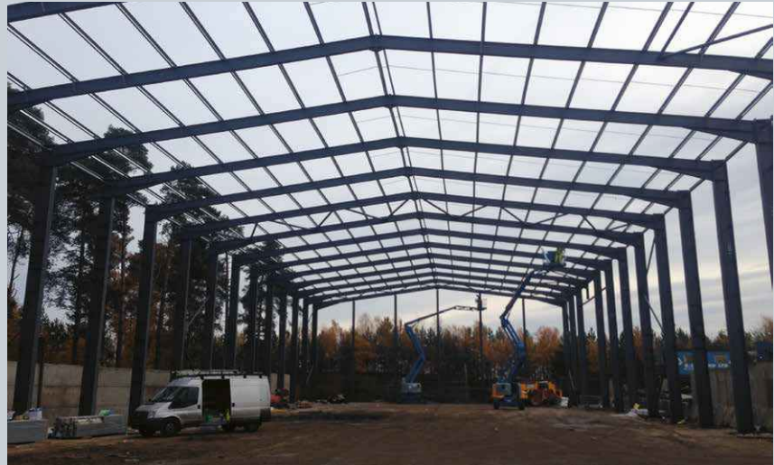
Opposite page: Robert Collard is on-site and the team receive the CIWM award from Nick Hewer. Above: the MRF structure uses waste metal. Below: the wash plant in action
